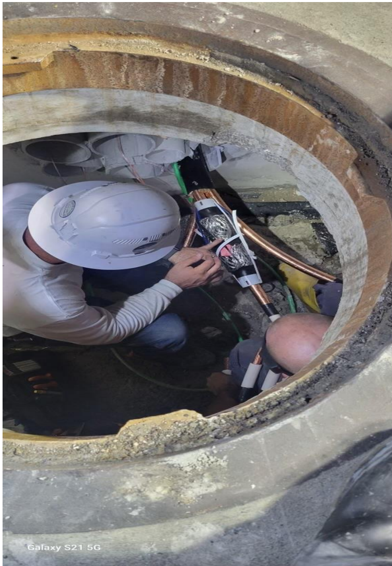
Figure 9- Cable splicing, Frank Matera
