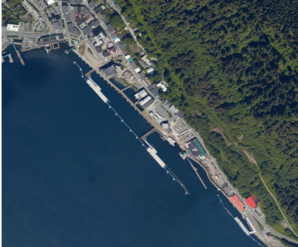
Figure 2- Port of Juneau's Cruise Ship Docks. Completed 2017. Matt Creswell
