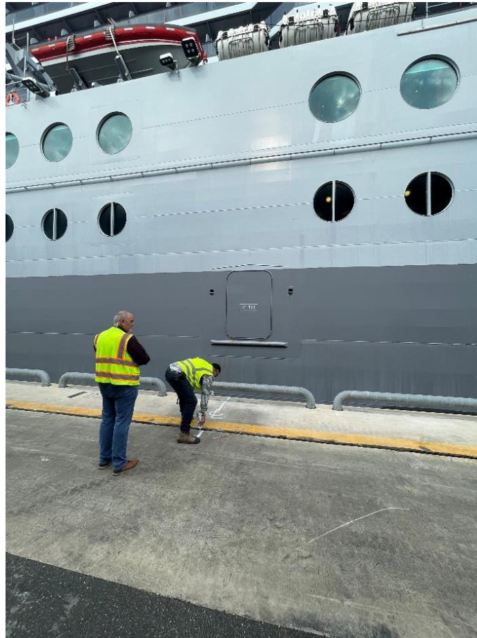
Figure 17- Frank and Armando measuring for proper fixed CMS placement, Matt Creswell
